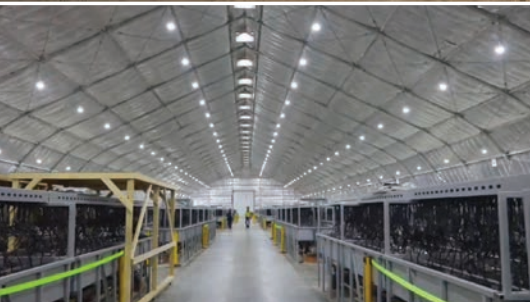
Large clearspan interiors
