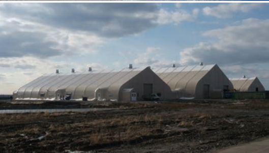
Remote processing facilities
