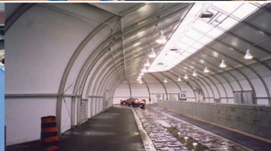
Daylight panels in peak create bright interiors
