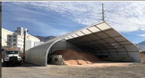
Sand and salt storage
