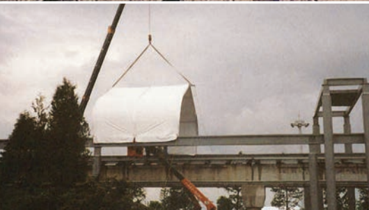
Remote processing facilities
