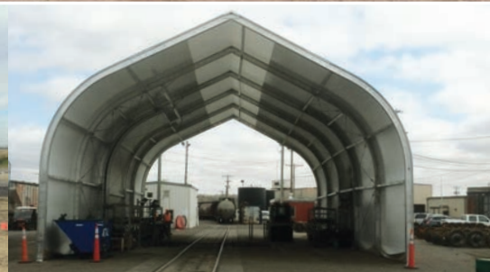
Large clearspan interiors
