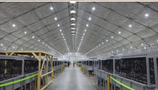
Spacious, clear-span interiors
