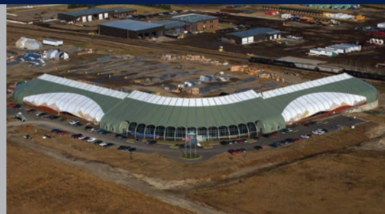
Office and distribution facility
