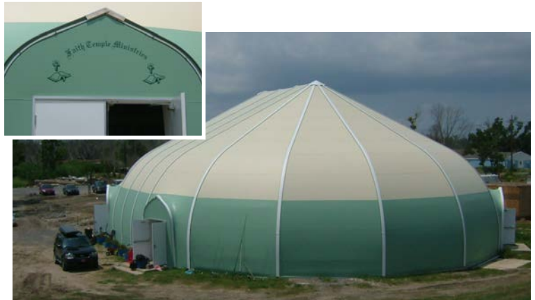
Exterior membrane replaced after Hurricane Katrina.
