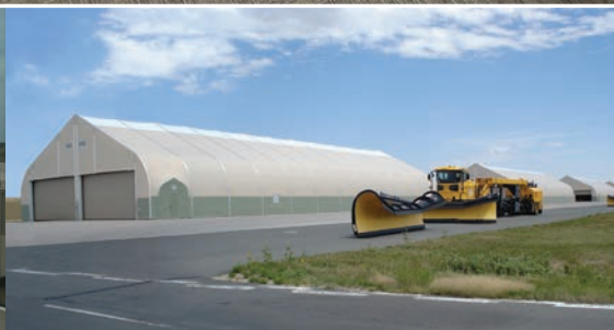
Snow removal equipment storage
