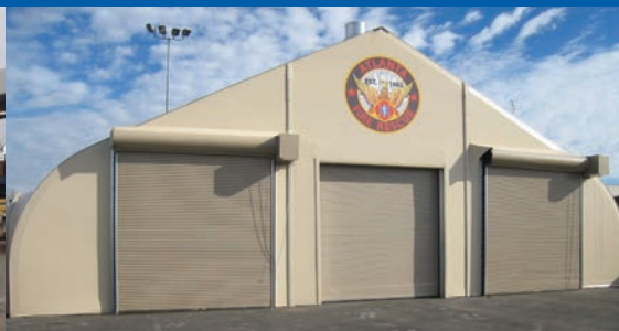
Emergency equipment storage
