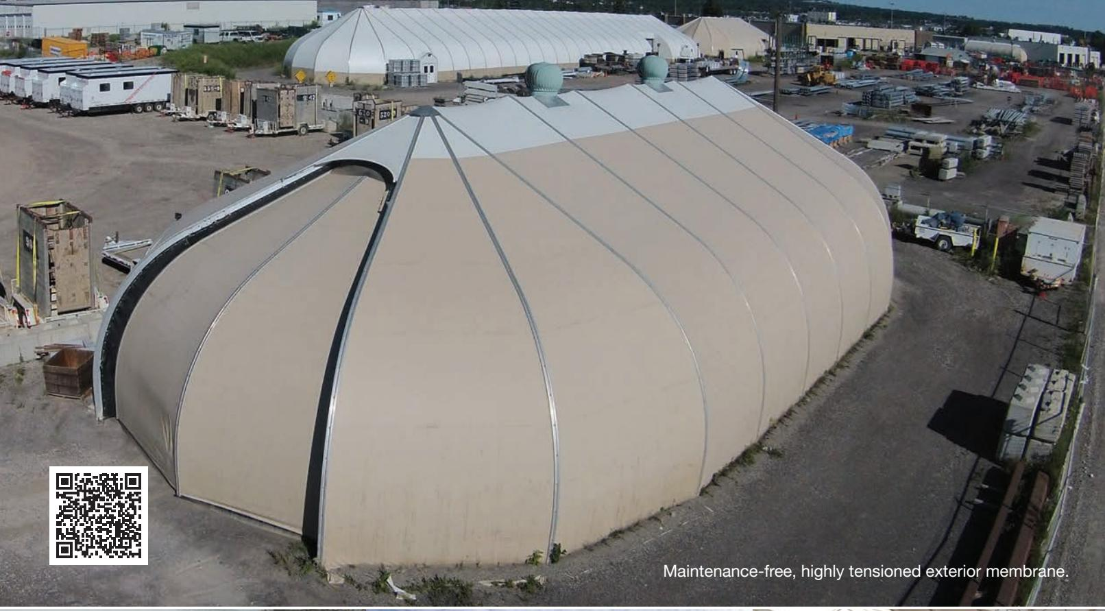
Maintenance-free, highly tensioned exterior membrane.
